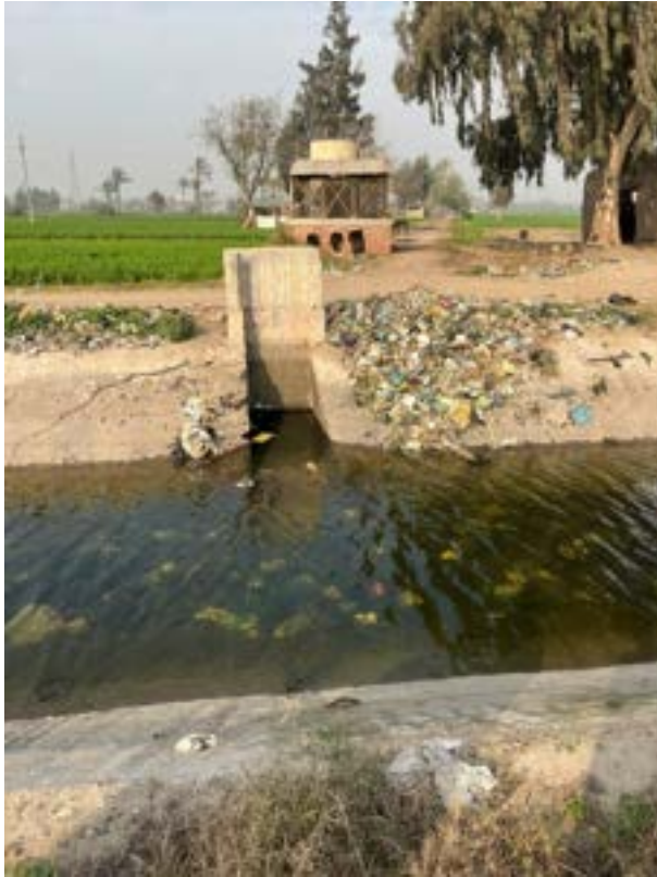
Figure 3.5 Poor condition of the concrete lining in the irrigation canal
