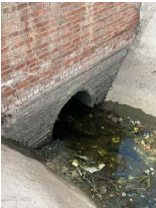
Figure 3.4 Outlet of the closed canal to the open canal towards the Buzoor Farm. Dimensions approximately 120x80 cm
