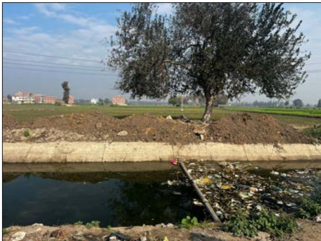
Figure 3 Ridges to stop water from the overflow
