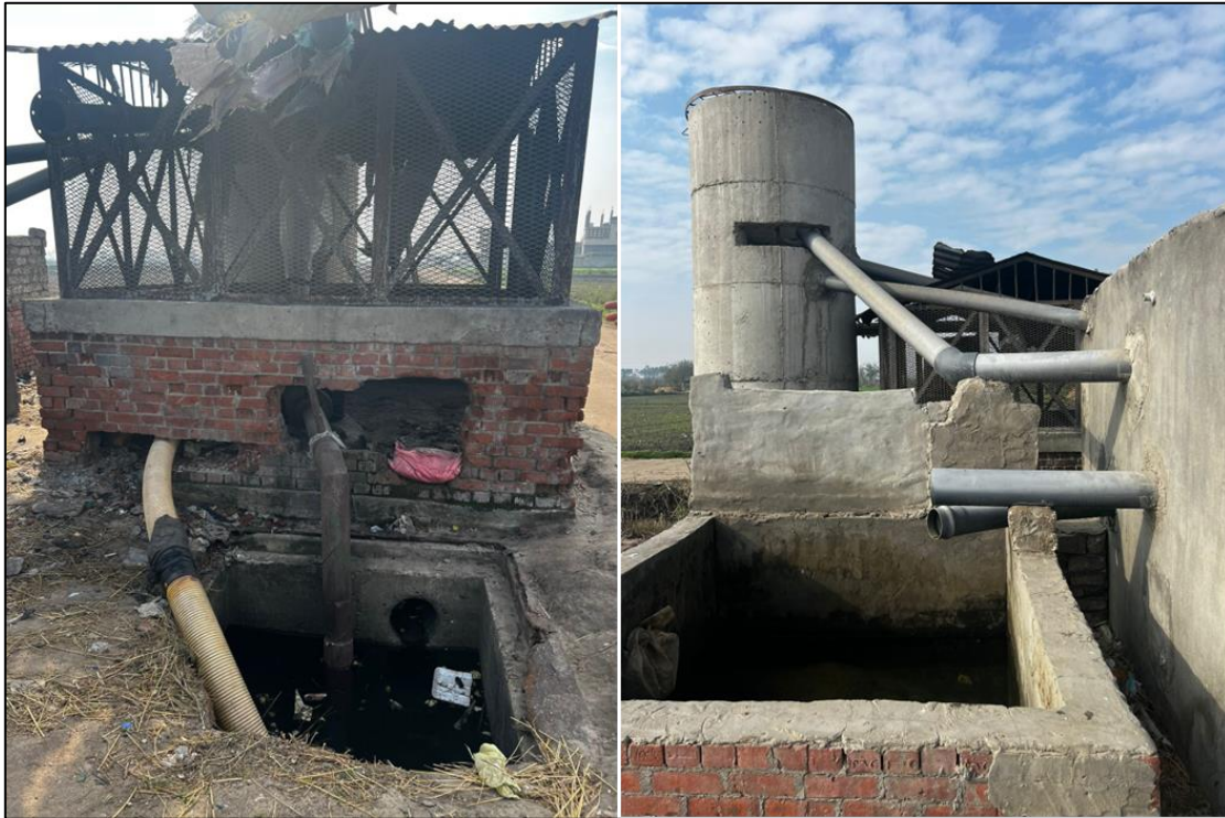
Figure 5 Improved Irrigation System (Governmental Project): Pump + Reservoir + Pipes + Valves
