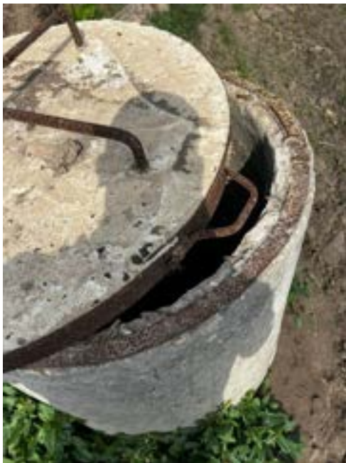
Figure 3.18 covered drainage system (not in use currently)
